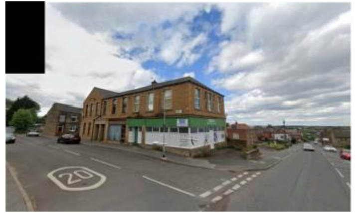
View of Site from Junction of Fountain Street and Elland Road
