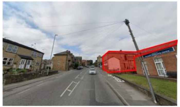
View from Elland Road looking South West
