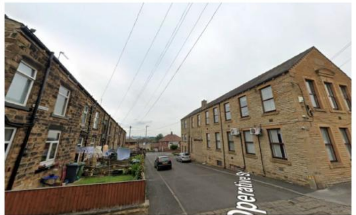
View looking down Cooperative Street
